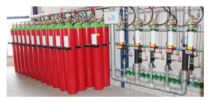
Equipment safe: Unlike many other agents that can become corrosive and permanently damage electronic components, Inergen does not form any corrosive by-products that can damage equipment in server rooms, data centres, medical facilities, laboratories or other sensitive electronic environments.
